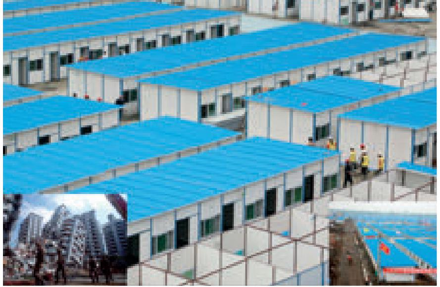
Fig. 2 - In 2008, in Sichuan (China), more than 1 million green prefabricated buildings were connected up with pipes for water, gas and electricity in the space of just 6 weeks
